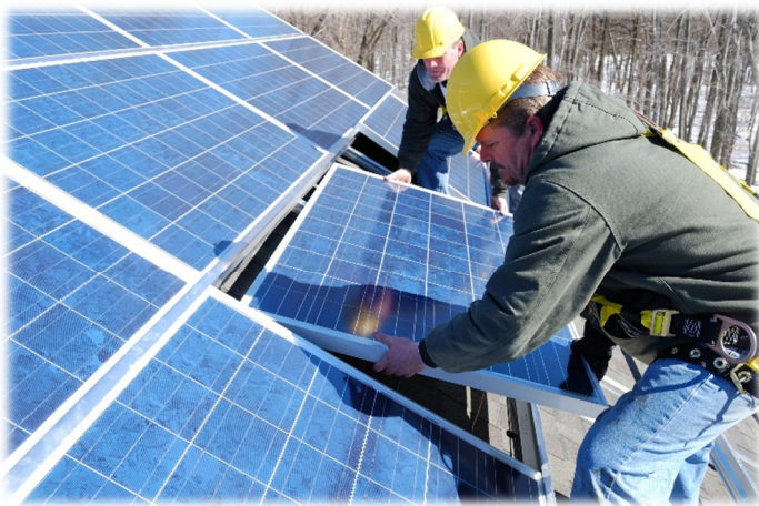
Tilt into place on the roof
